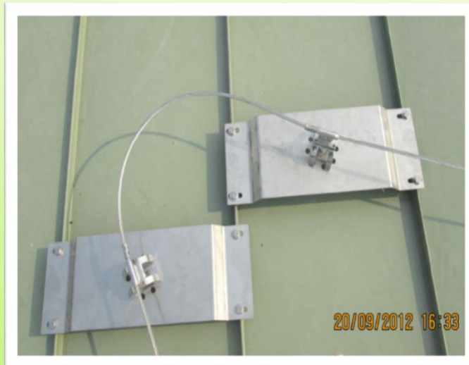
Figure 6: Curved Section on a Standing Seam Roof
